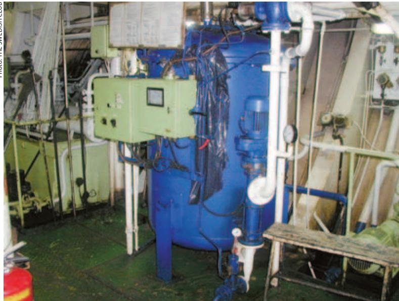
*An Oily Water Separator is not enough – the layout of the bilge systems and holding tanks must be appropriate.*
