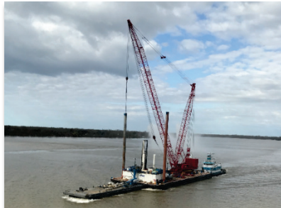
Photo 8: Typical crane and/or deck barge assistance
